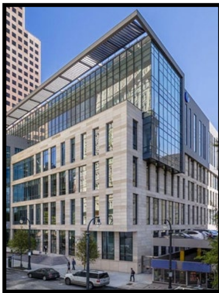
Figure 2 The Mix Apartments
