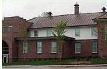
Bessie Strong Hall Opened 1917 Renovated 2004 Capacity 10 Headcount 10
